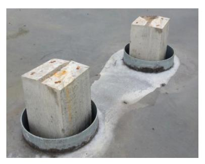
Note The piles are largely decoupled from floor slab loading but probably worth preloading before use
