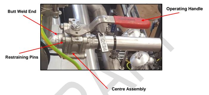
As defined by their use, each value is directly positioned into the water circuit. The section of circuit containing the value must be isolated and the pressure relieved / coolant drained before working upon the value. To replace a complete centre section or to replace the seals, refer to sketch above and proceed as follows:
