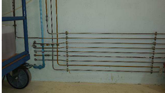
Figure 5 : Possible attachment of the distribution and return lines inside the accelerator tunnel.
