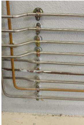
Figure 5 : Possible attachment of the distribution and return lines inside the accelerator tunnel.
