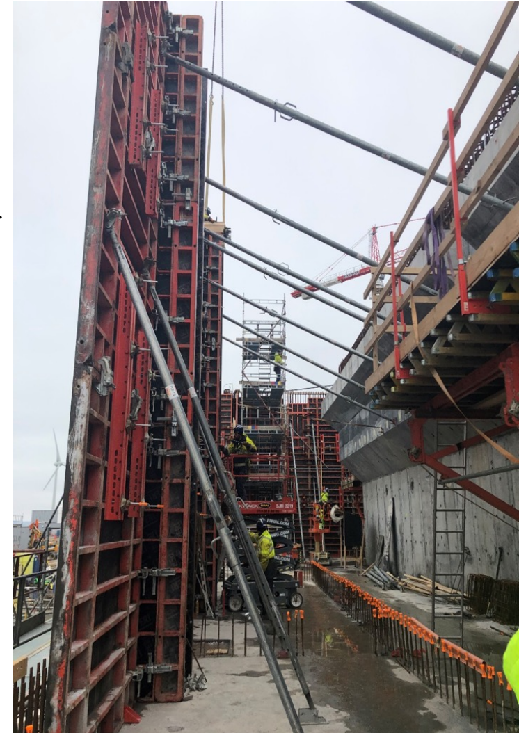
Forms for Technical Gallery walls
