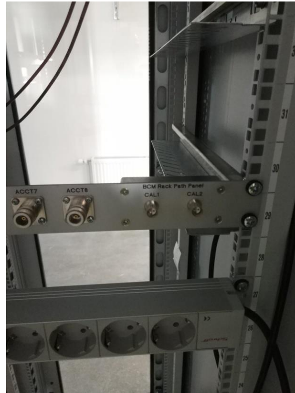
BCM patch panel from rack no. FEB-050ROW:CNPW-U-013 and BCM patch box
