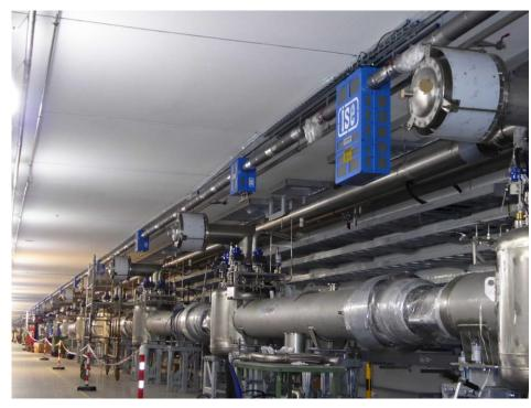
Distribution of 2 frequencies (352.21 MHz and 704.42 MHz) from MO to the tunnel Total length: ~600m. Number of taps: 58 No of outputs: 294 Power level at each tap: +17 dBm Stability requirement: 0.1° for short term(during pulse 3.5 ms)
