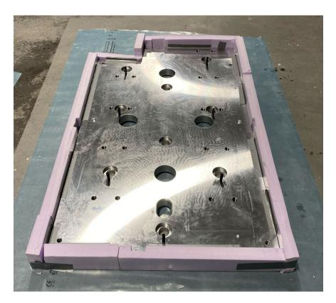
Baseplates rigging and preparation for grouting : Foamwork – tape – grease
