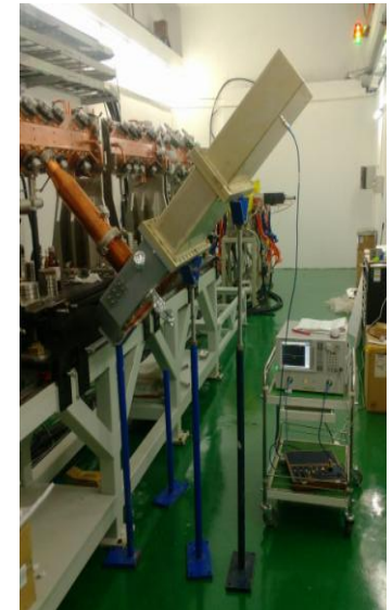
Coupler installation on RFQ
