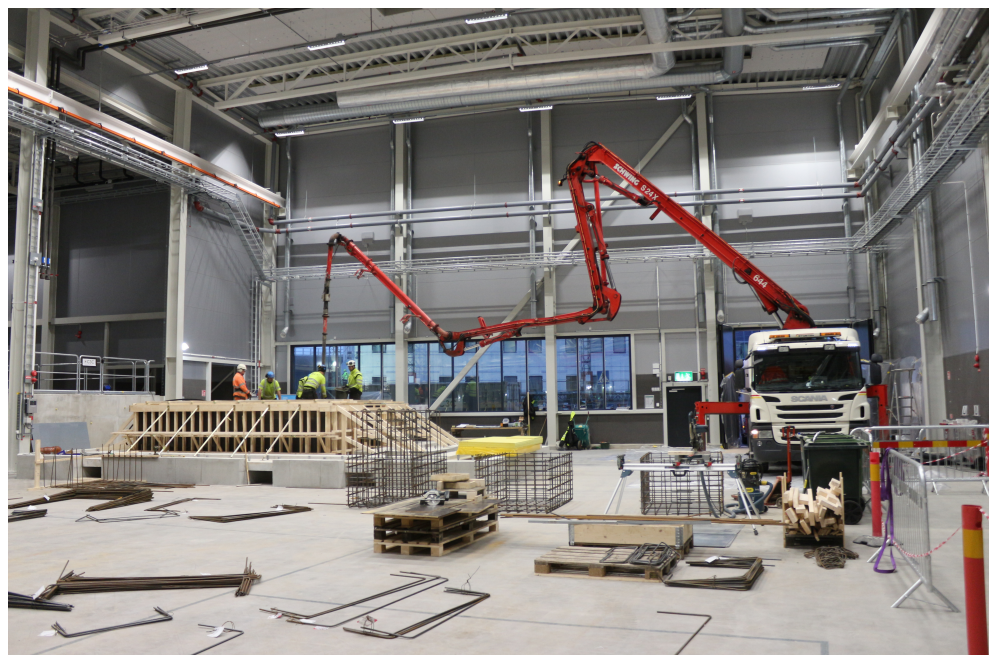
Figure 2 Access and space needed changed during different phases
