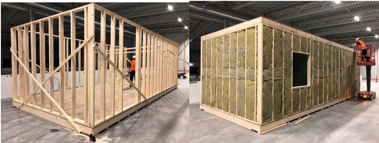
Figure 7 – Build progress showing structure (left) and with additional insulation (right)
