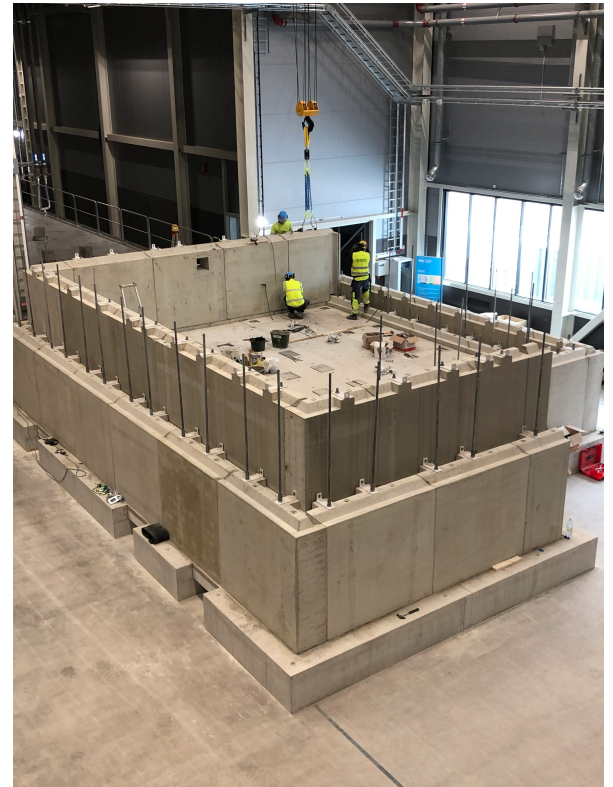
Figure 1 Crane operations at NMX Cave
