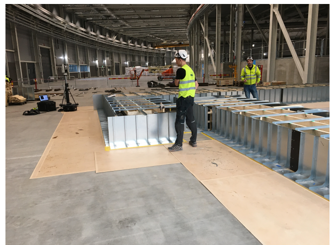
Figure 4 Metrology operations verifying walls positions
