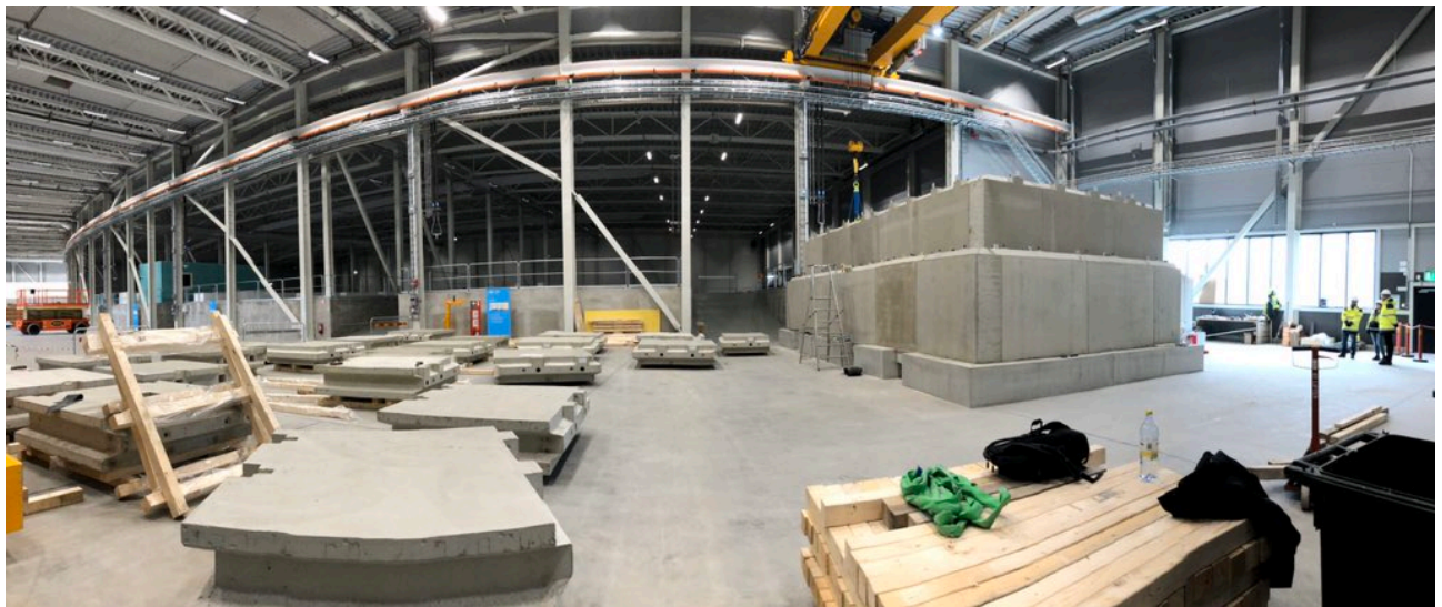
Figure 3 Logistic needs were agreed with area coordinators
