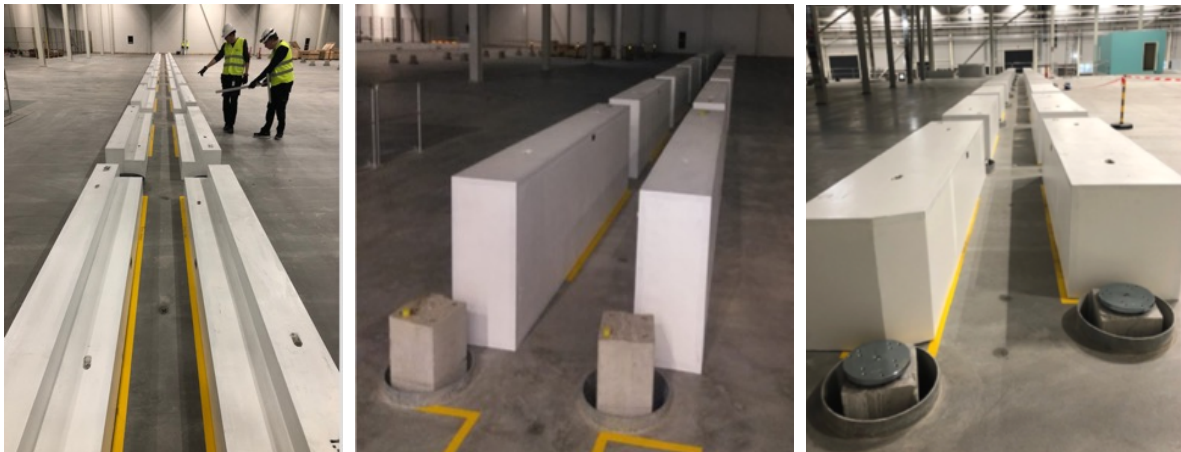
Figure 3. Left: MAGIC lower blocks installed in E02:1, Dec 2019. Middle: BIFROST lower blocks installed in E02:1, Jan 2020. Right: CSPEC lower blocks installed in E02:1, Feb 2020.
