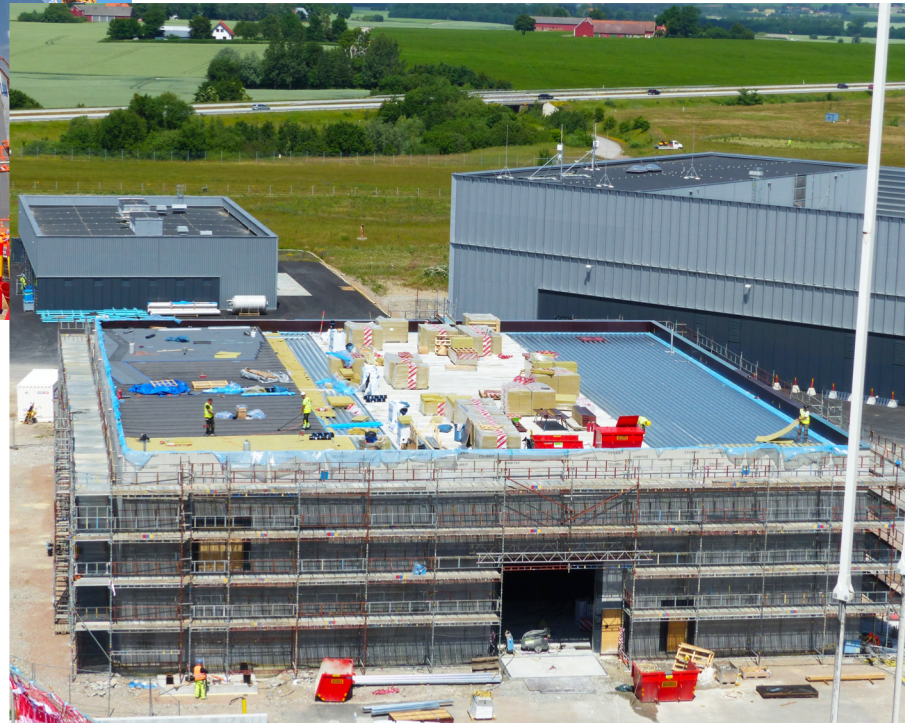
Roof works completed in H09 Radwaste
