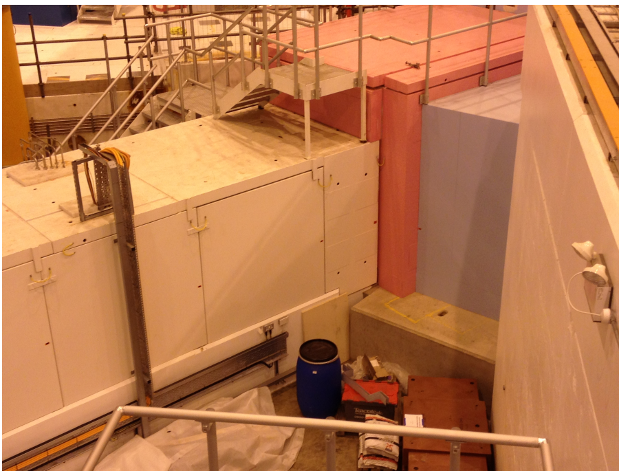
Figure 5: A step in the shielding support floor to reduce ground-shine. This example is partially covered by the wooden panel. The step is in the white concrete base, near to the orange blocks.
