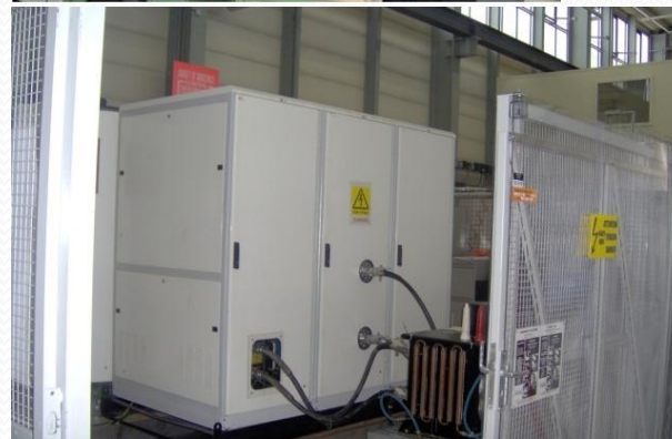
100kV RRCAT modulator during acceptance tests at CERN.
