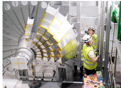
Installation of endcap detectors
