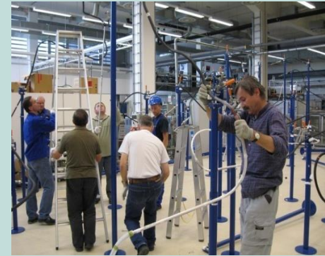
Handling of the bus bars in the preparation area
