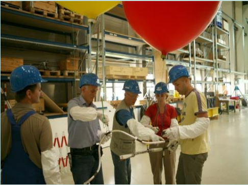
Transportation of a single bus bar to the preparation area
