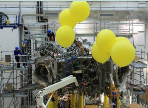
Installation of the bus bars on the module
