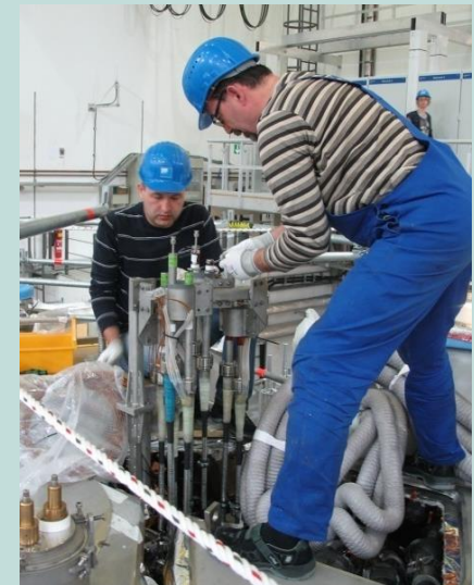
Clamping of the bus bars to the structure
