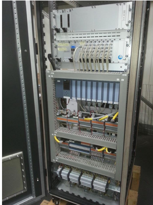
Instrumentation cabinets for M-ECCTD control
