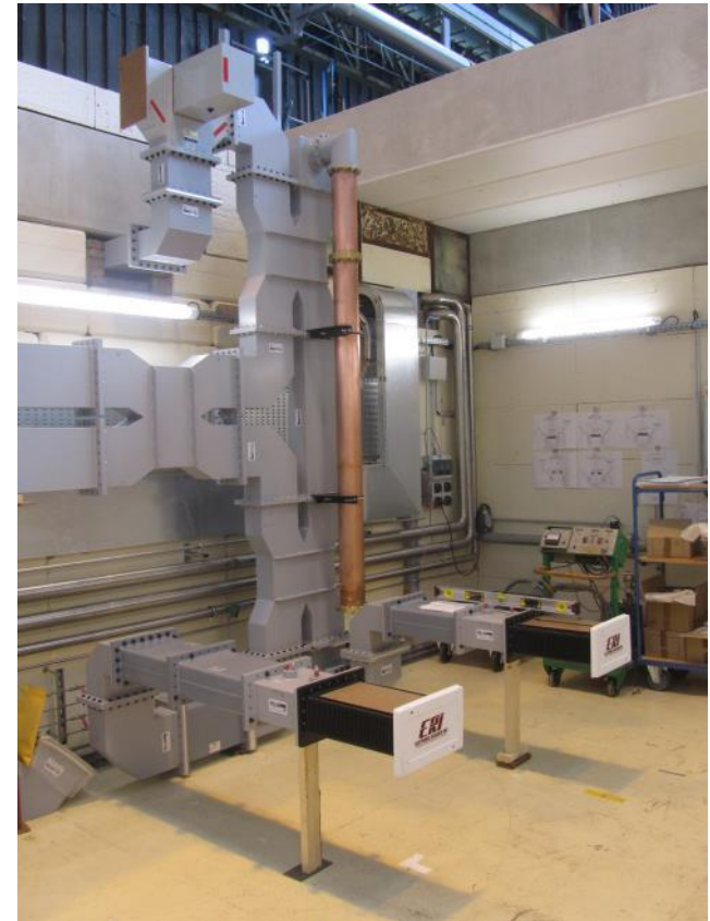
RF distribution (Installation in progress)
