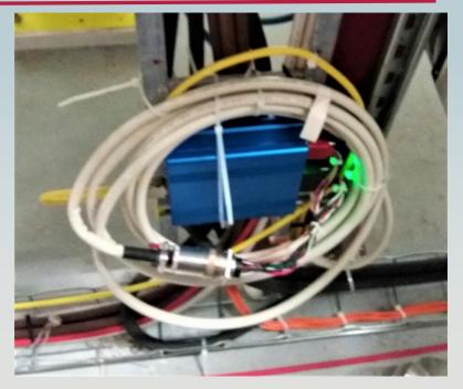
The complete WS ACQ system has been moved and installed on LINAC4: µ-TCA and VME crates + **Back End Analog Front End** in LINAC tunnel
