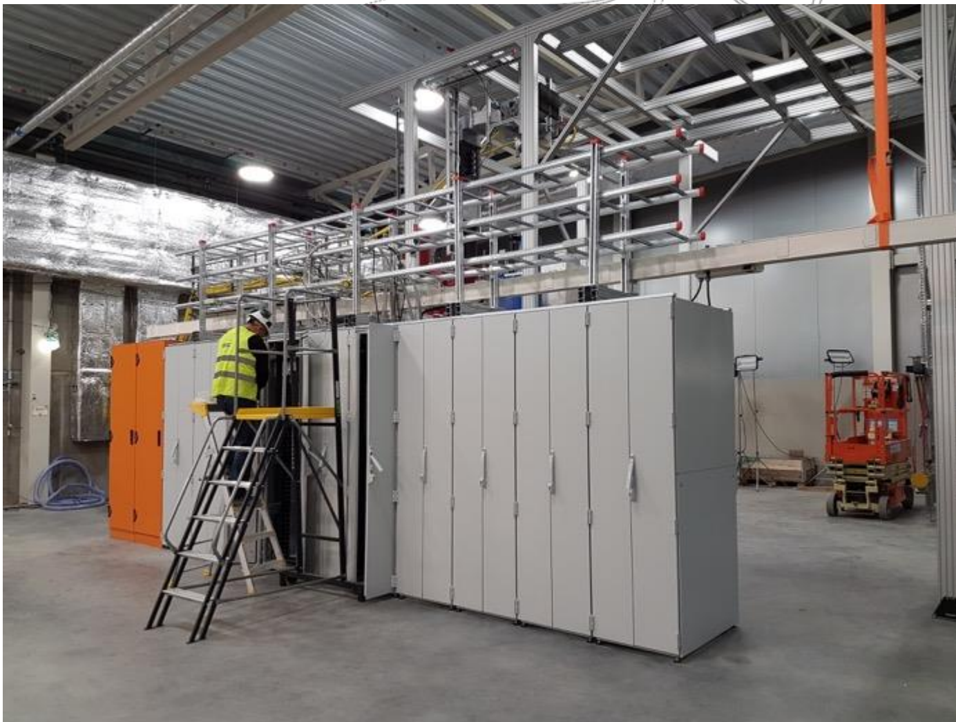
Installation of Racks, Cable Trays and Power Distribution
